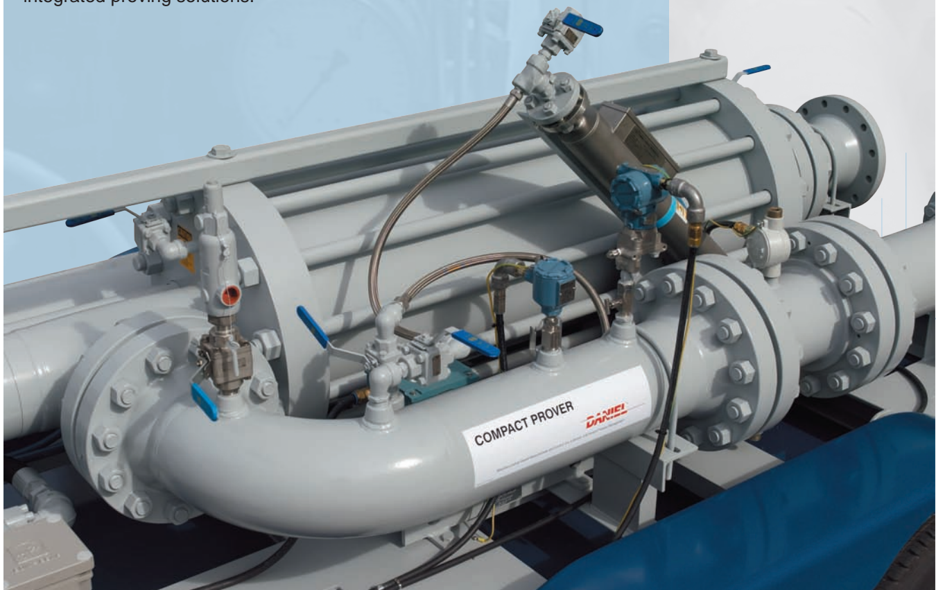
Compact Prover with Liquid Turbine Flow Meter and Fast Loop Densitometer
