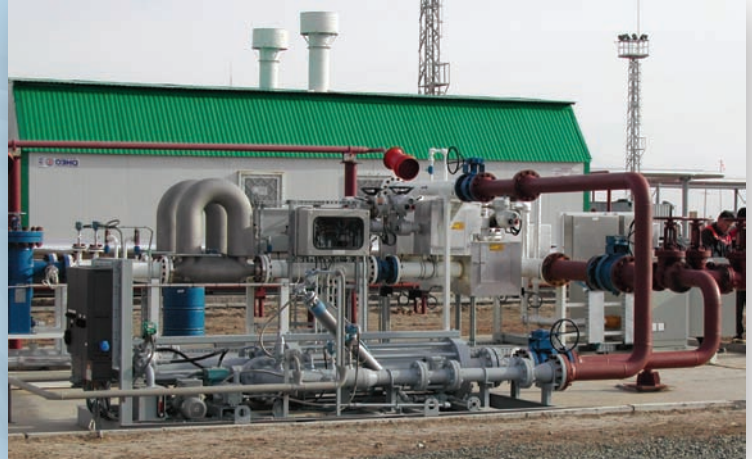
Compact Prover proving Coriolis flow meters on a mass basis
